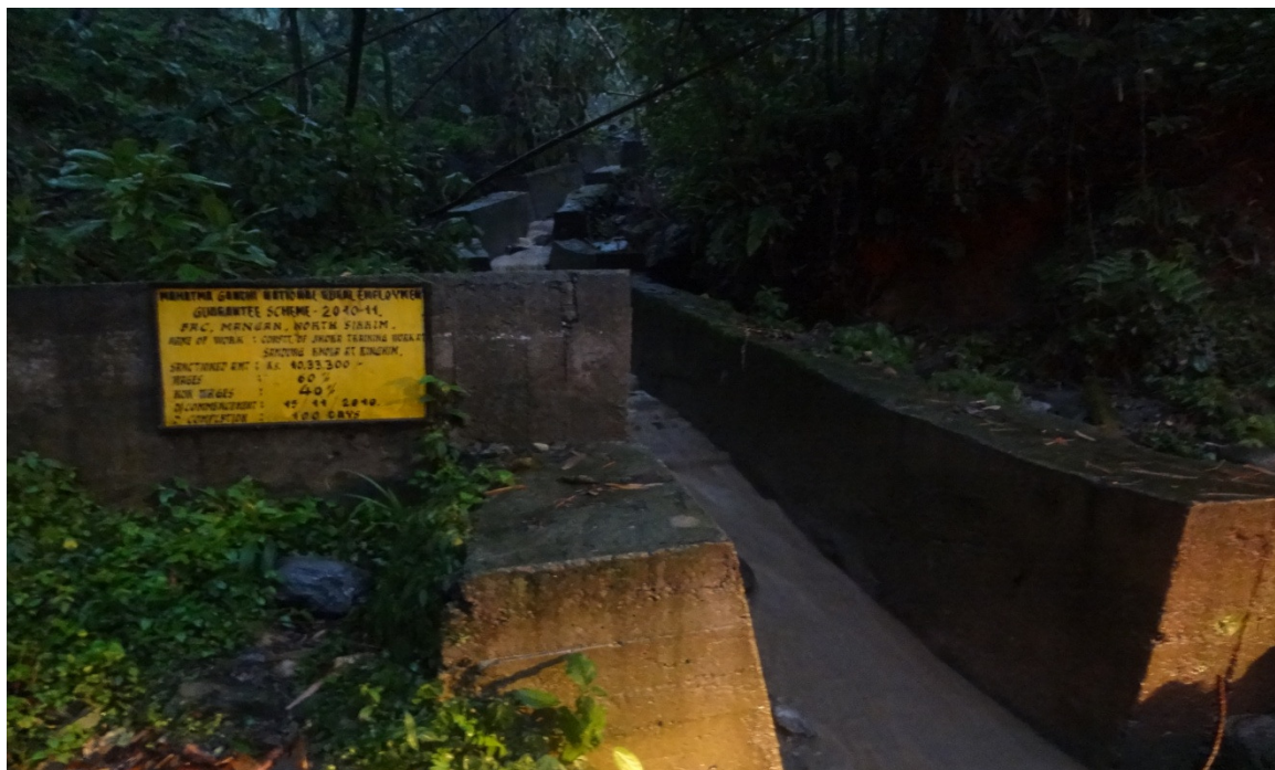
Drainage System Constructed under MGNREGA, Village-Ringmim, BAC-Mangan, North Sikkim
