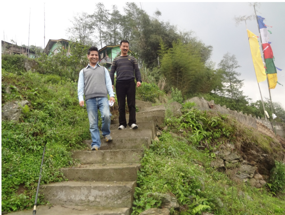
Habitation Connecting Road constructed under MGNREGA, Village-Namok Sheyam, BAC-Mangan, North Sikkim
