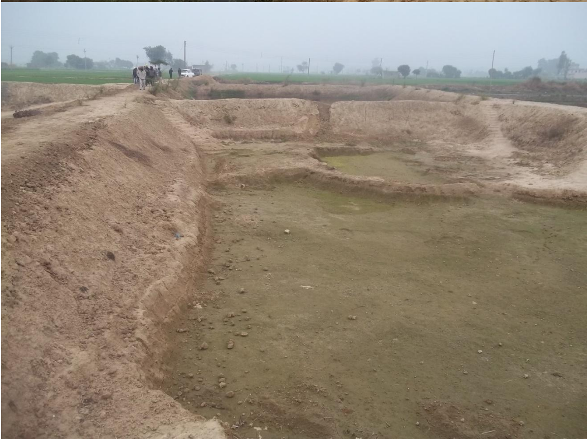
Photographs after Partial Completion of work
