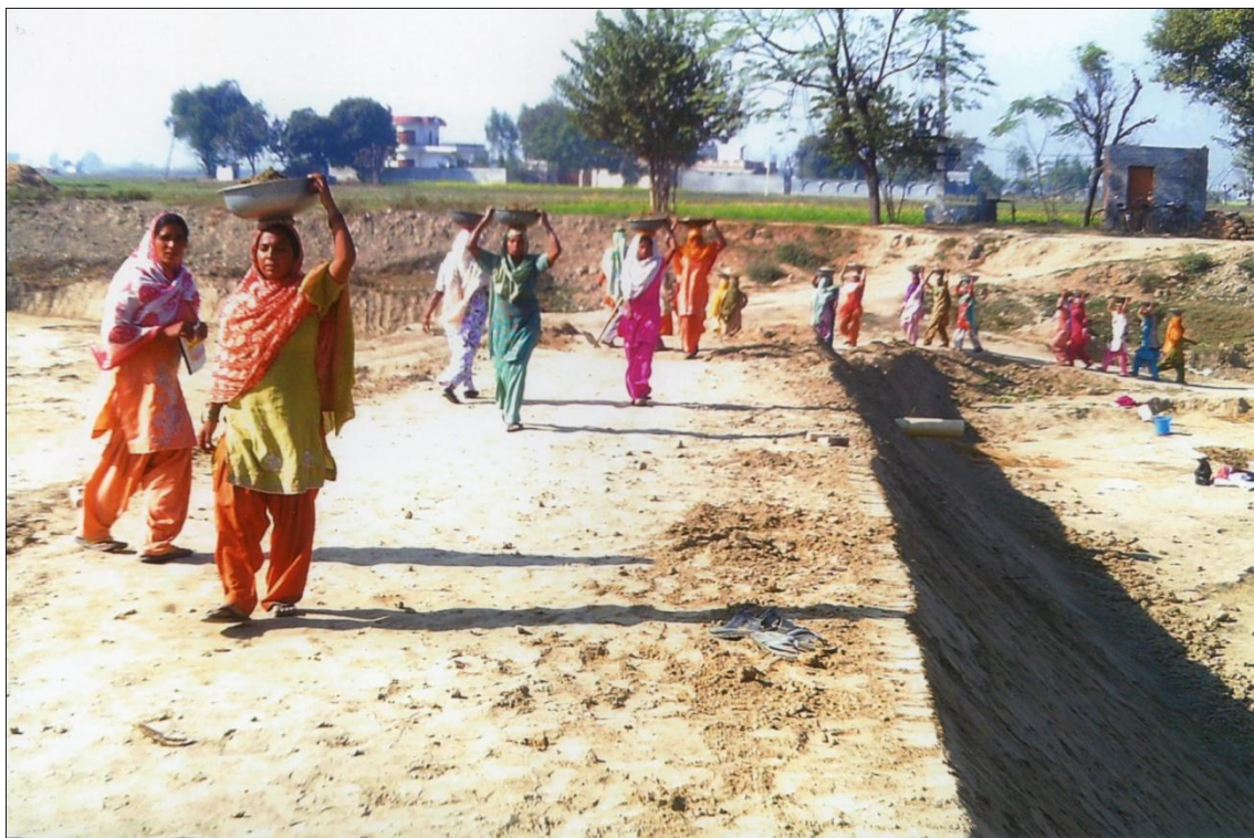
Work in Progress under MGNREGA
