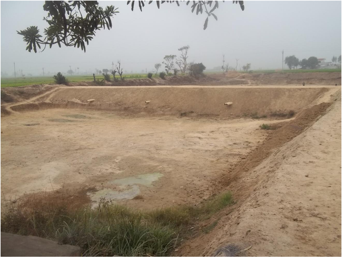
Photographs after completion of work of two chambers
